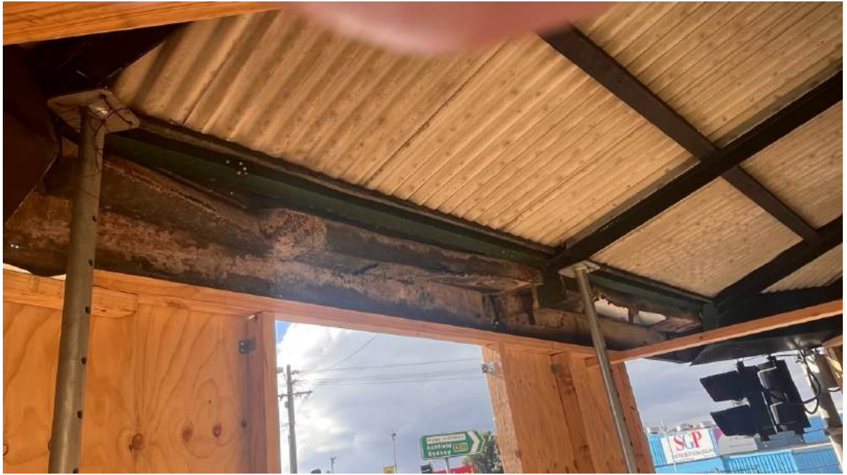
Fig.16 Corroded guttering
