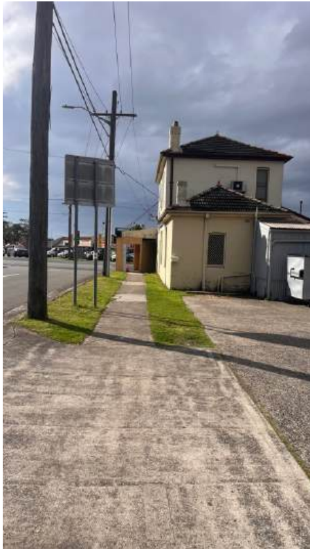
Fig.9 Site and awning from Meredith St.
