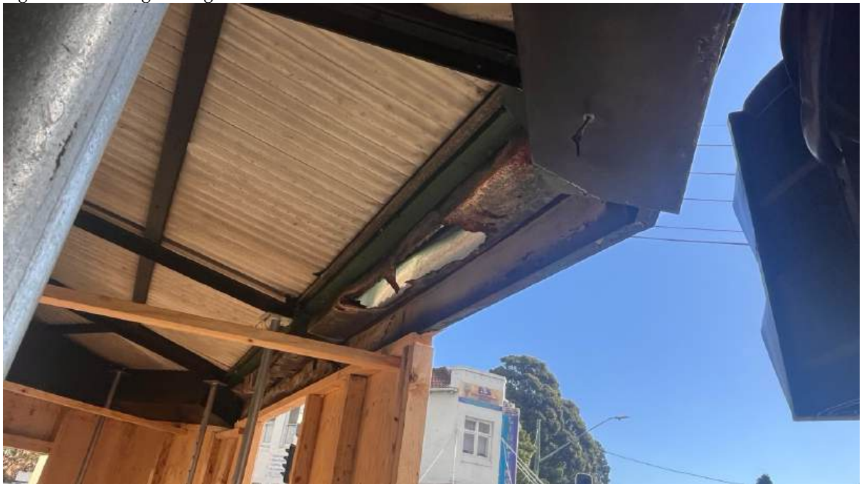
Fig.17 Corroded guttering
