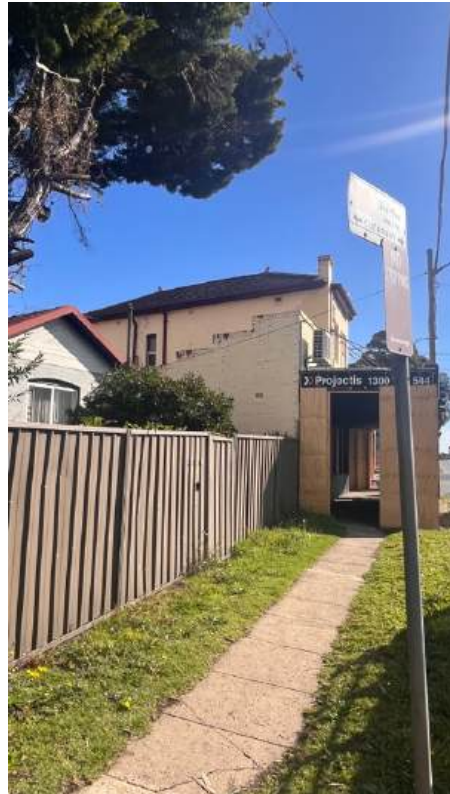
Fig.19 Subject site from Hume Highway
