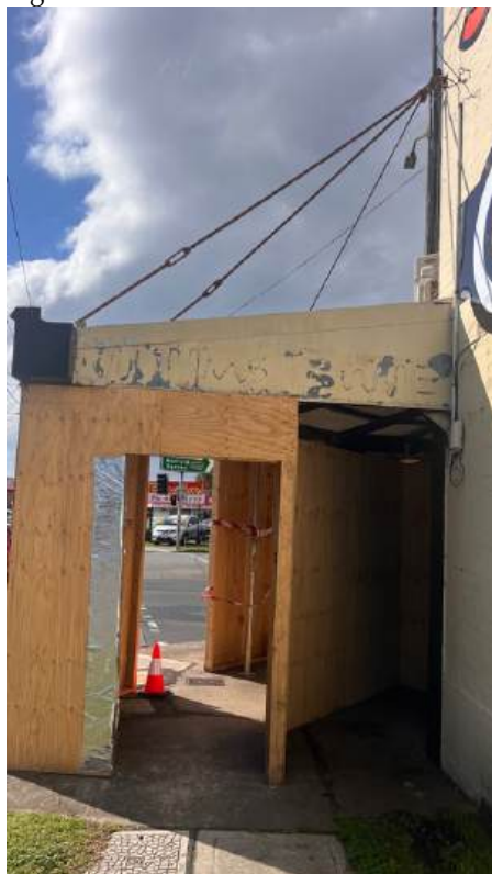
Fig.12 Site and awning from Meredith St.
